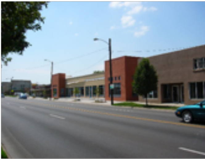
East Grand Avenue Master Plan and retail development by the Neighborhood Development Corporation, Des Moines.
